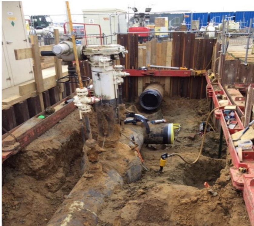
Figure 6: Bacton Terminal excavated valve.
